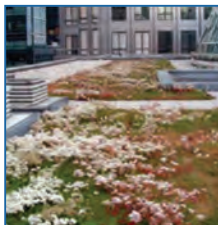
Sedum roofing system
